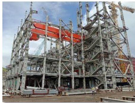
Main Building Installation
