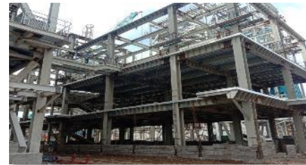
Central Control Building Construction
