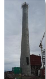
Chimney Concrete completed
