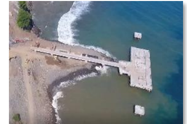
Coal Jetty progress
