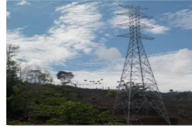
Transmission tower completed
