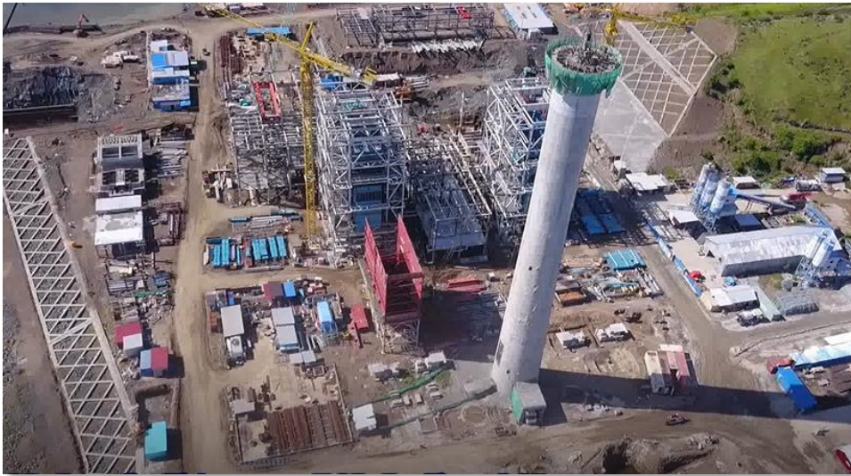
Site Condition (Main Plant)
