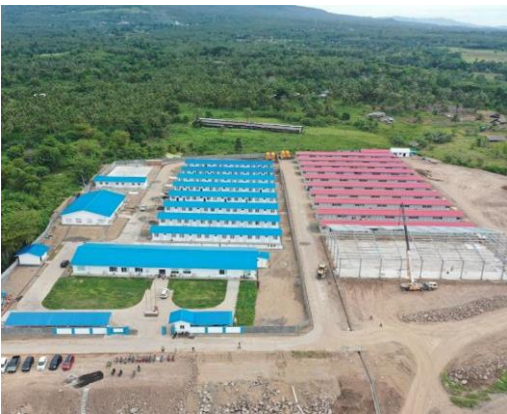
Camps & Temporary Warehouse
