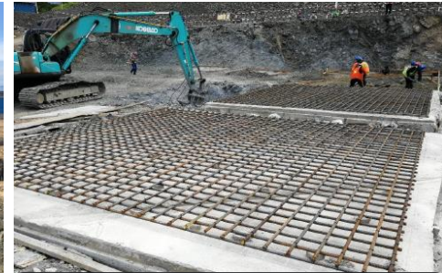
Steel reinforcement in foundation
