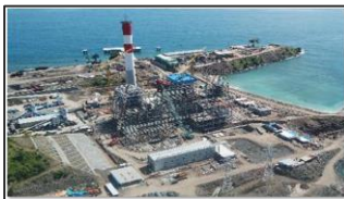
GLP Main plant
