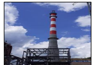
MCL Chimney Construction
