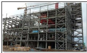
GLP Main Building Installation
