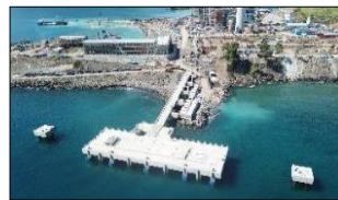
GLP Coal jetty construction
