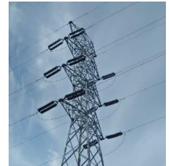
Cable Stringing Finished
