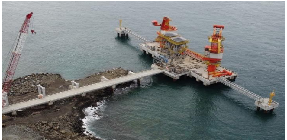
Coal Jetty and Coal Handling System progress
