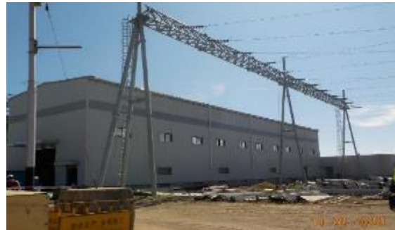
150 kV GIS room progress
