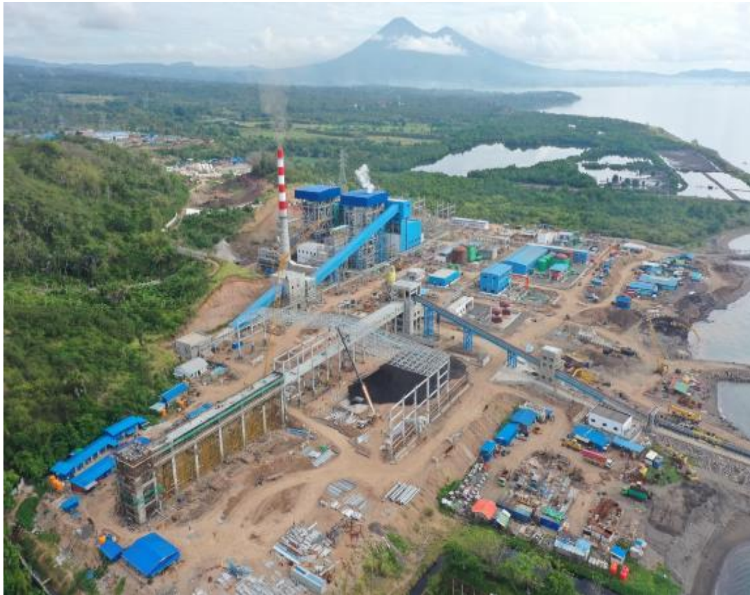
Main Plant Overview
