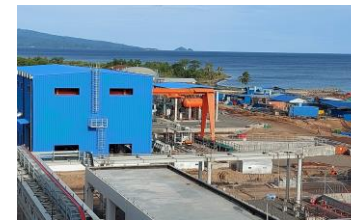
Water Pump System
