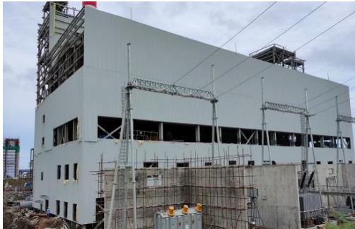
Main Building Installation
